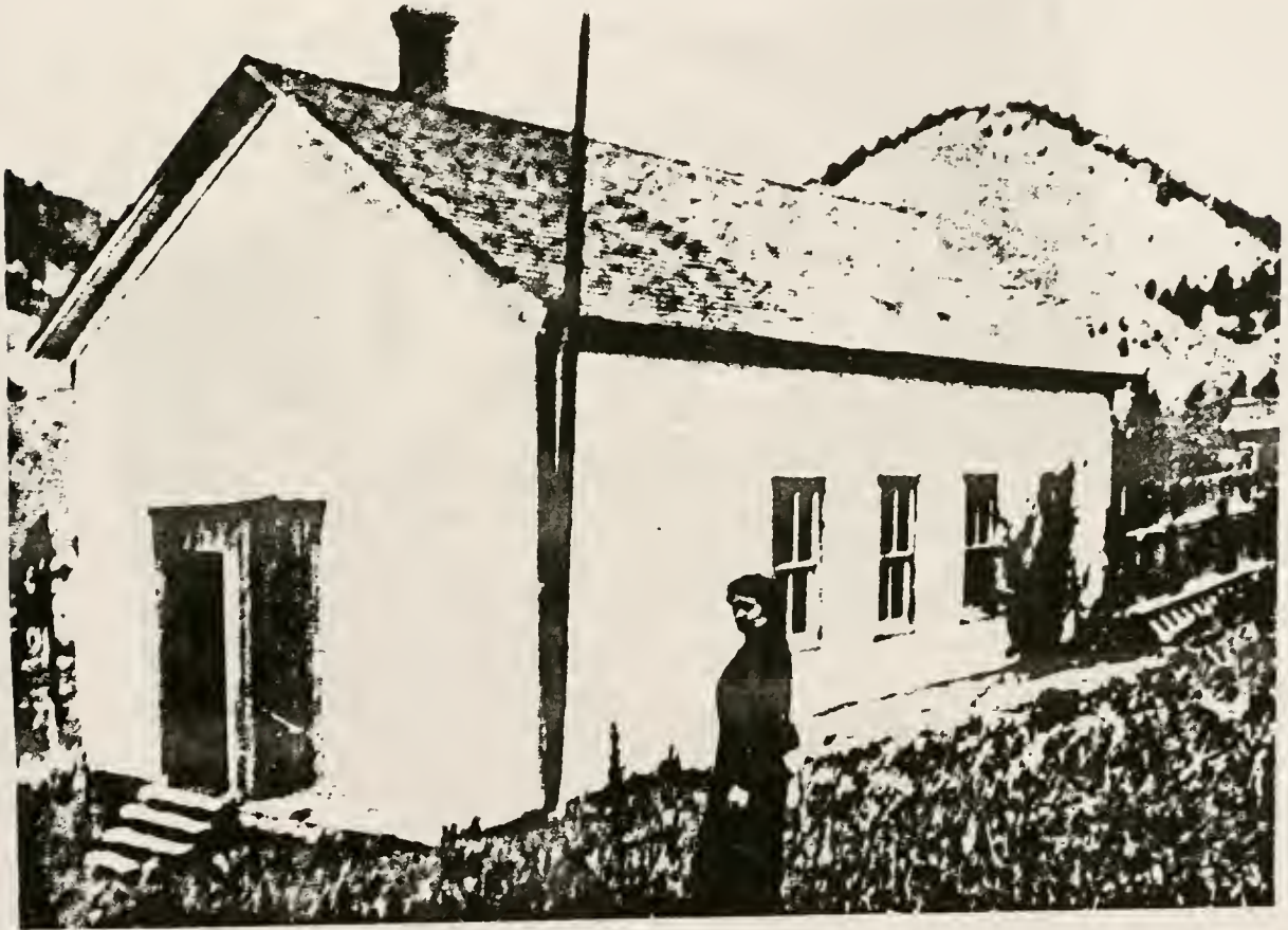
Figure 203. Jardine school house (Structure #79). Photograph ca. 1910-1920, Courtesy of Bill and Doris Whithorn. Park County Museum, Livingston, Montana.
